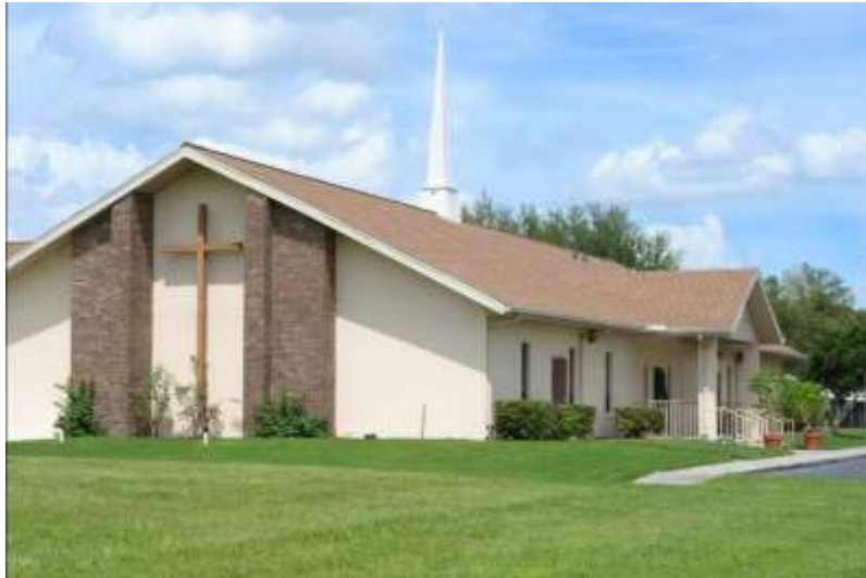
Orlando Central Baptist Church
