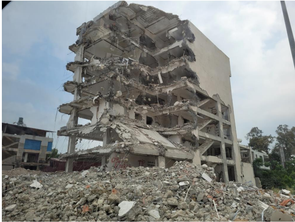
Damage in Antakya from the Earthquakes in February 2023
